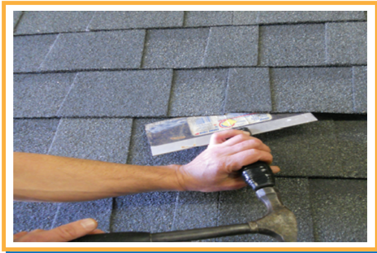
Figure 13. Lifting Shingles for Installation of Heating Panels
